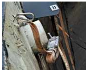
Figure 5: Belt package fixed with cable tie – located directly next to mixer mast. Belt fixed at wall. Snap hook for fixing net
